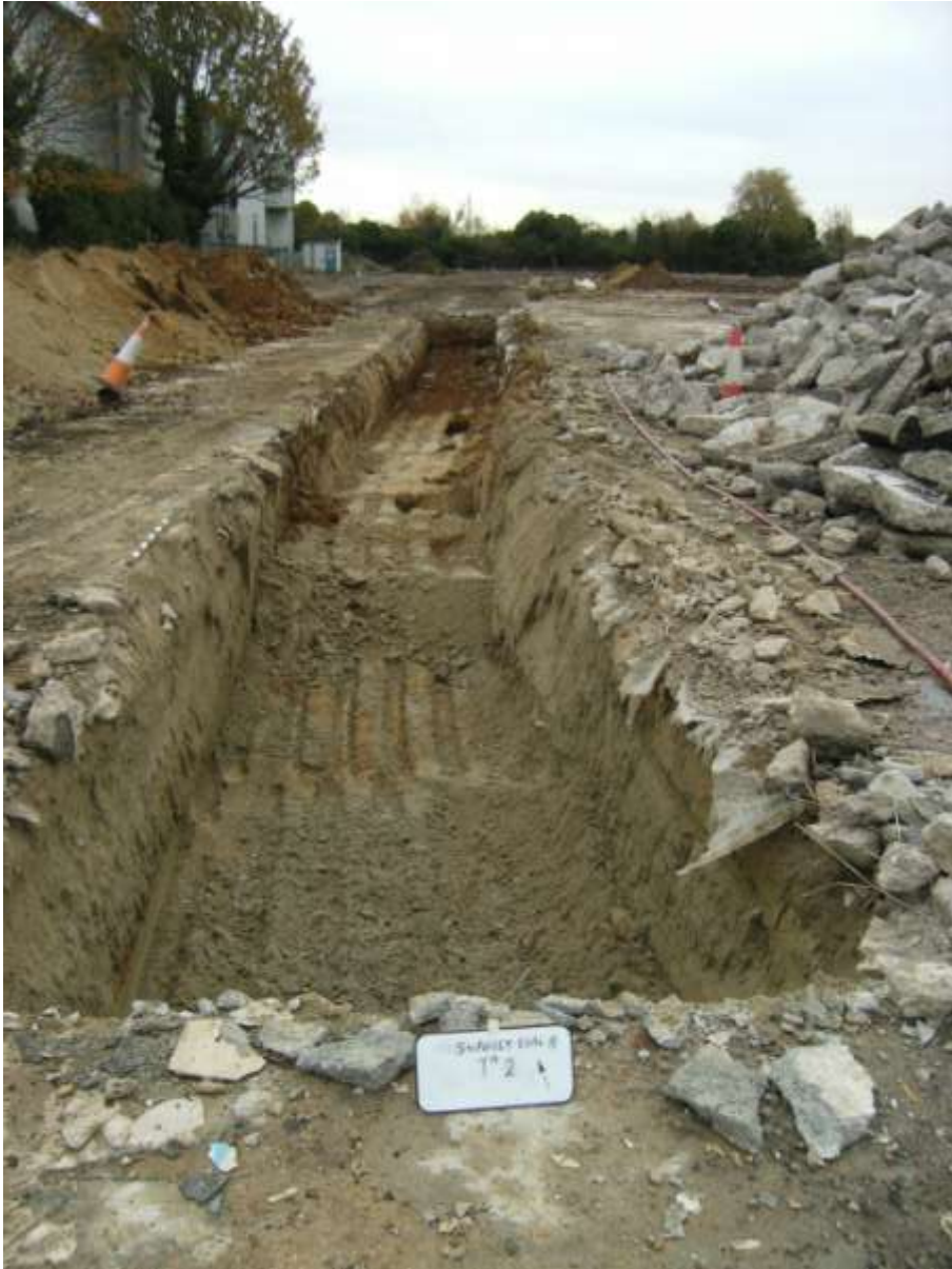
Plate 5 – Trench 2 (looking NE)
