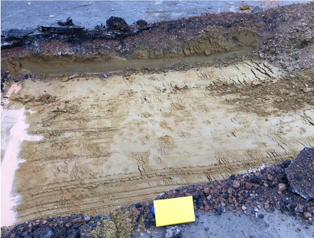
Figure 9: Trial Pit TP8 photograph, Goldsel Road, Swanley, Kent. Trench depth here is 0.40m.
