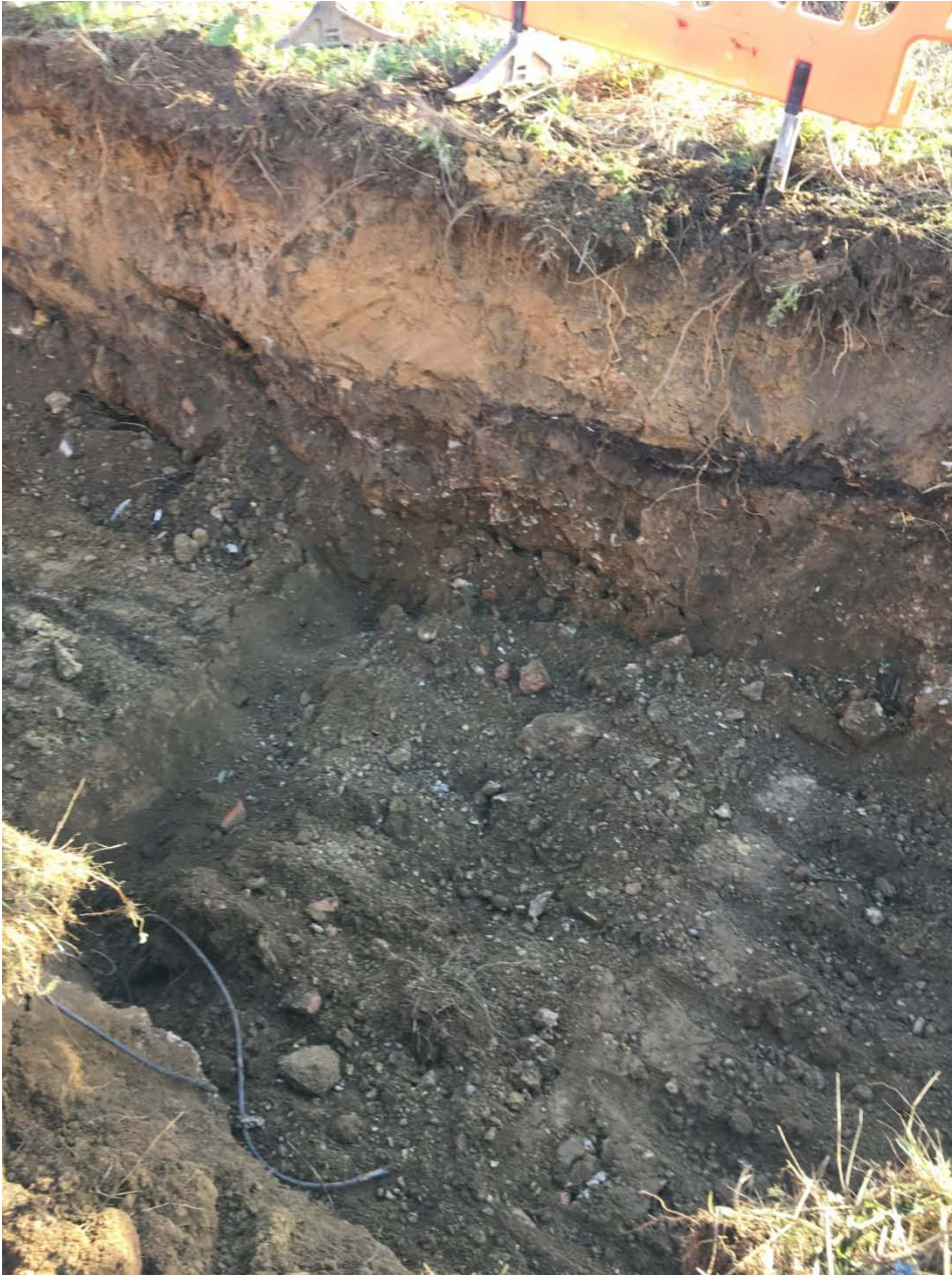
Figure 8: Trial Pit TP7 photograph, Goldsel Road, Swanley, Kent . Trench depth here is 1.2m.
