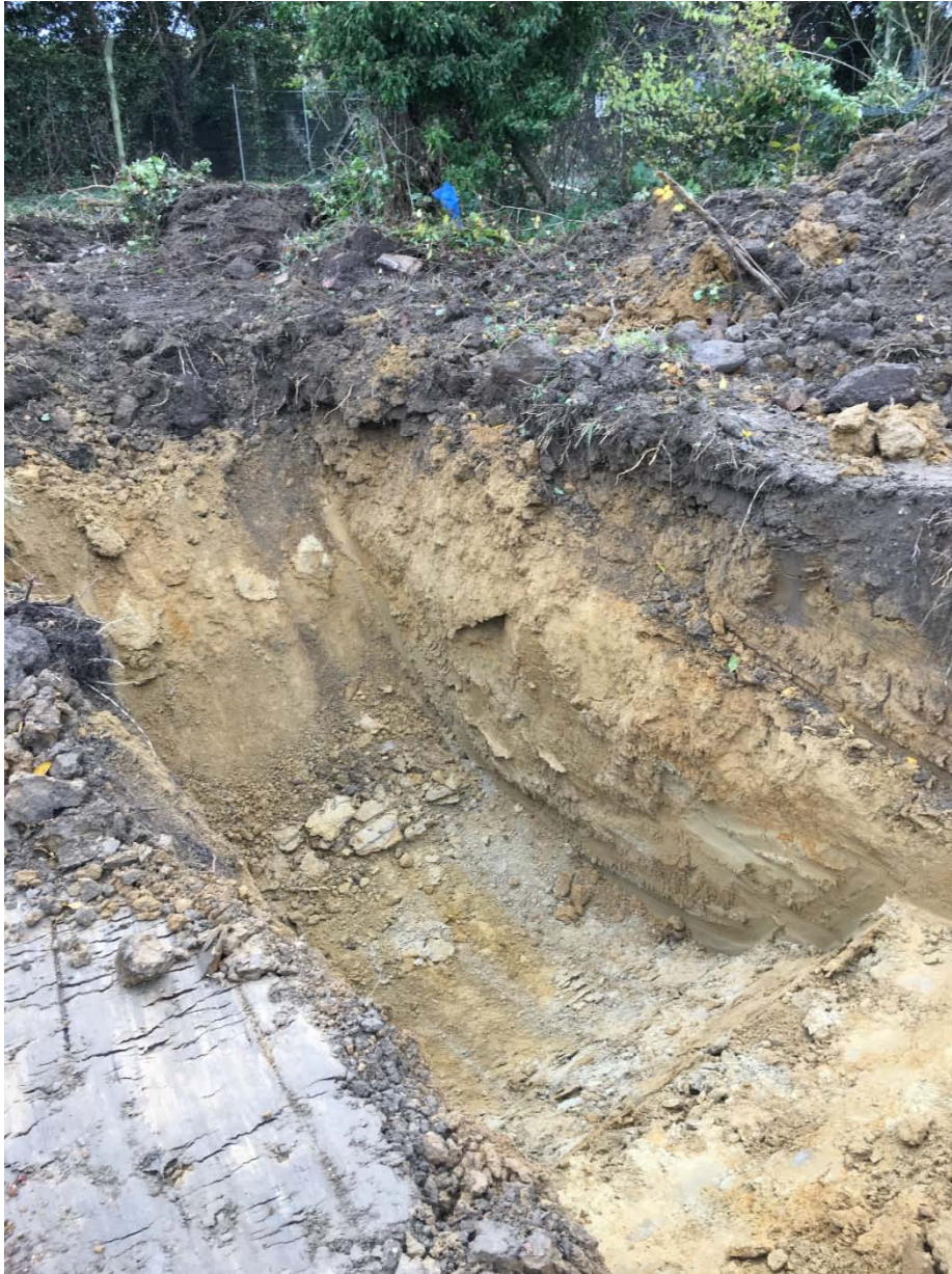
Figure 11: Trial Pit 10 photograph, Goldsel Road, Swanley, Kent. Trench depth here is 2.30m.
