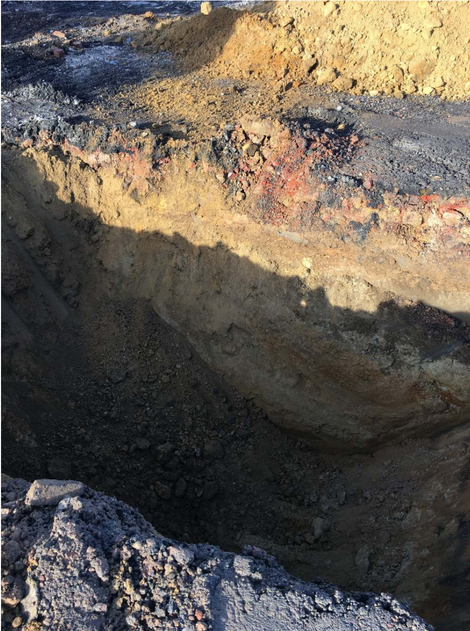
Figure 6: Trial Pit TP4 photograph, Goldsel Road, Swanley, Kent. Trench depth here is 1.5m.
