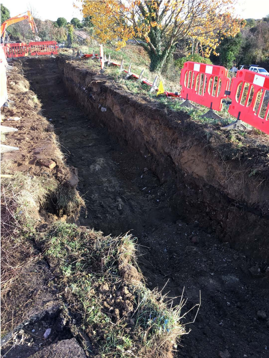
Figure 7: Trial Pit TP5/6 photograph, Goldsel Road, Swanley, Kent. Trench depth here is 2.0m.
