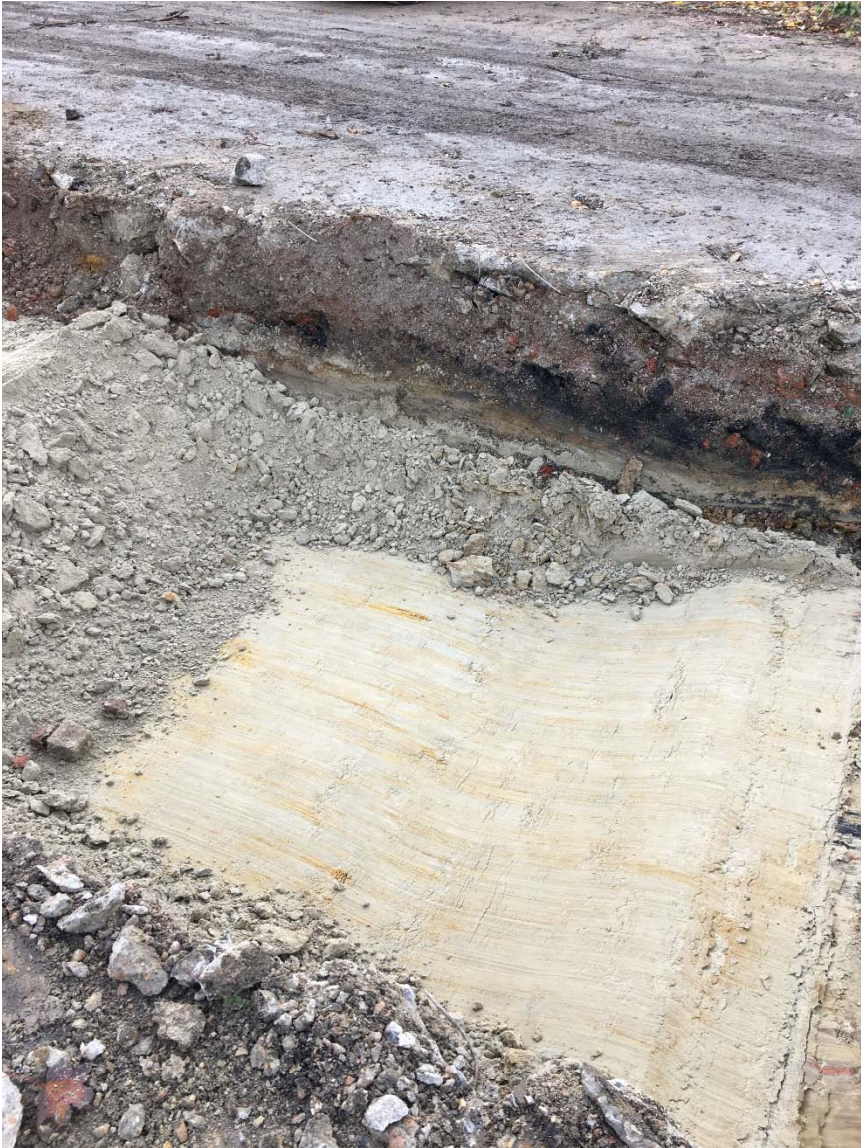
Figure 5: Trial Pit TP3 photograph, Goldsel Road, Swanley, Kent. Trench depth here is 0.5m.
